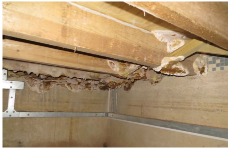
Left, top: Dry-rot fungus Left, below: Insect infestation (woodworm) Right: Thatch, lime plaster and limewash: Aberdeunant, Llansadwrn
