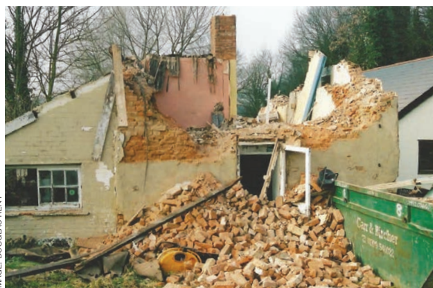
Lime mortars allow the reuse of bricks following demolition.
