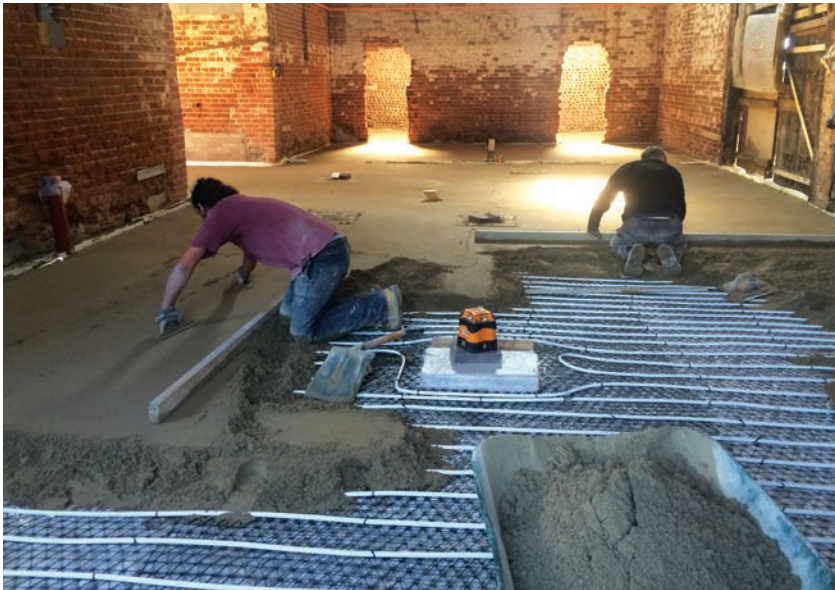
Cork insulating render during application. Left: A limecrete floor, incorporating underfloor heating, is laid.
