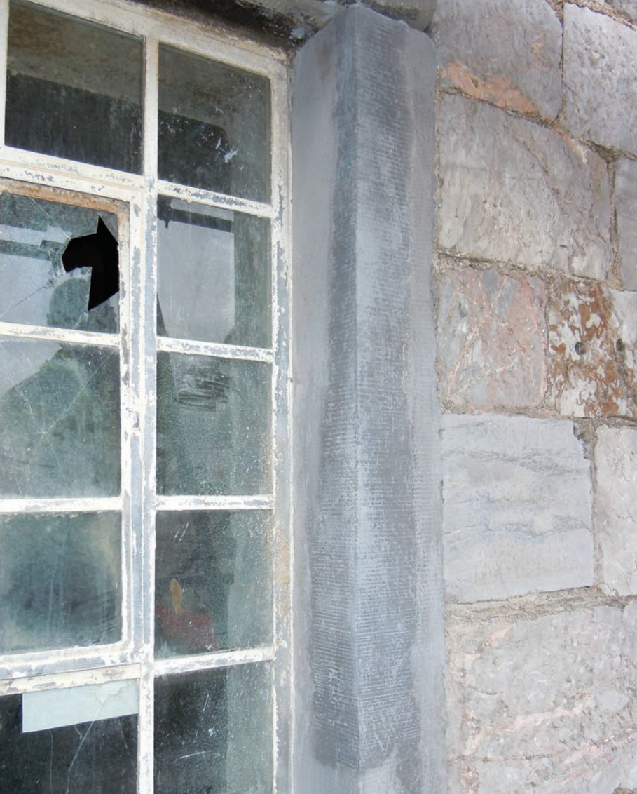
Left: Tile and mortar repair to window jamb. Below: Jamb before repair. Opposite: Stonework at Temple Church, Bristol, after conservation.
