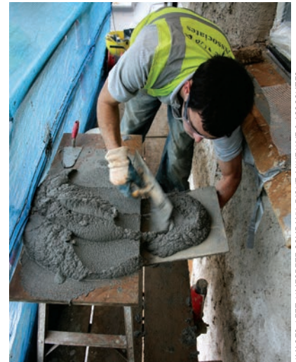
Cork insulating render during application. Left: A limecrete floor, incorporating underfloor heating, is laid.
