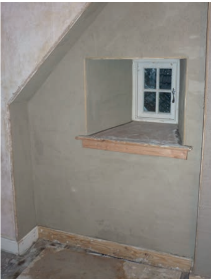
Fig. 6 Plaster applied to laths in large scale repair.
