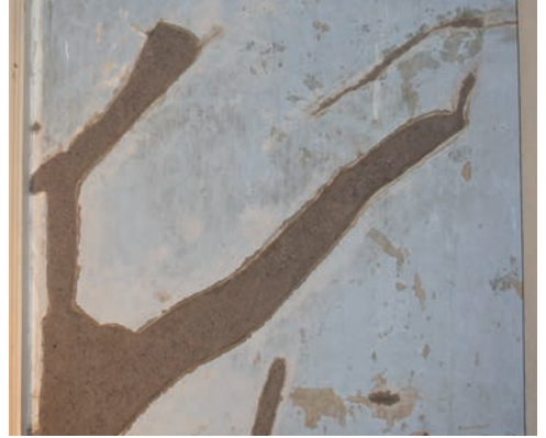
Fig. 8 First coat of coarse plaster used in a patch repair.
