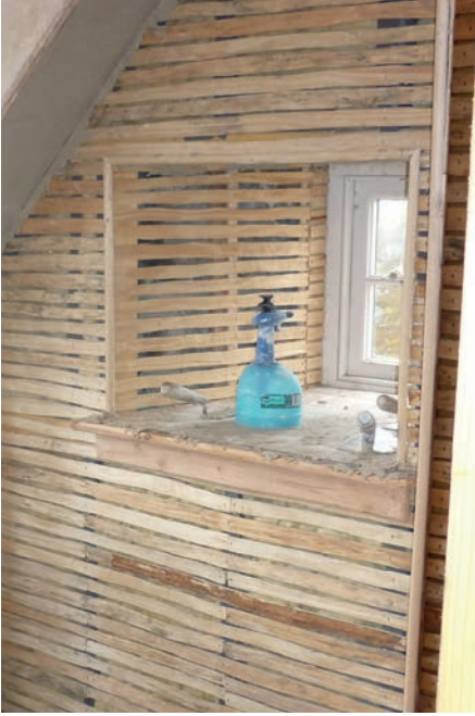
Fig. 5 Replacement timber laths ready for application of base coat.
