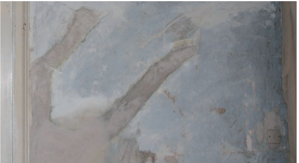
Fig. 9 Finishing coat applied to patch repairs ready for decoration when the plaster has set.
