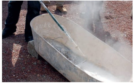
Fig. 1 Quick lime being slaked using traditional methods.
