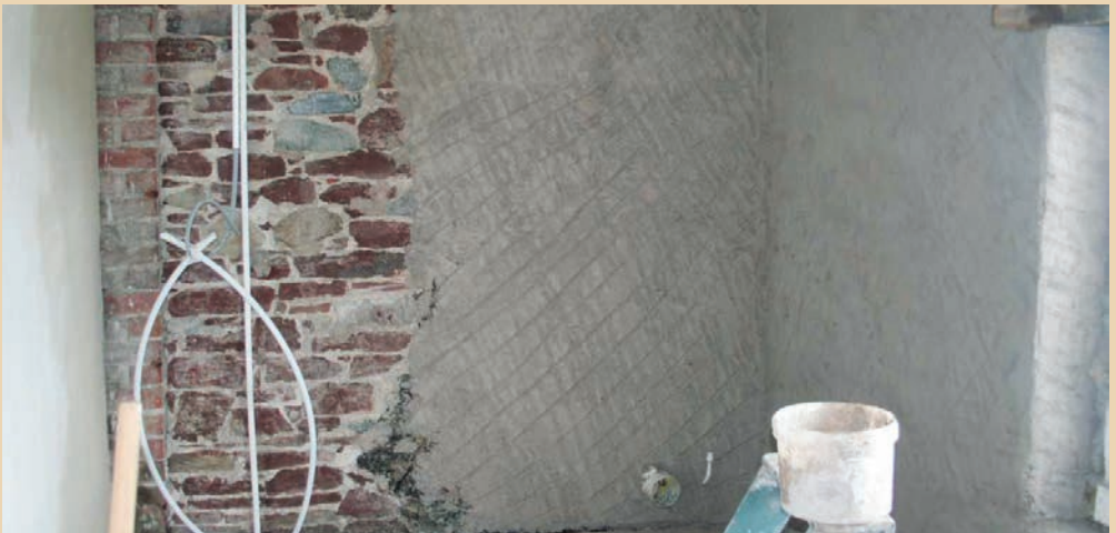
Fig. 4 Scratch coat of plaster applied on the hard directly to a rubble masonry wall. (Photo credit: Eden Hot Lime Mortars)
