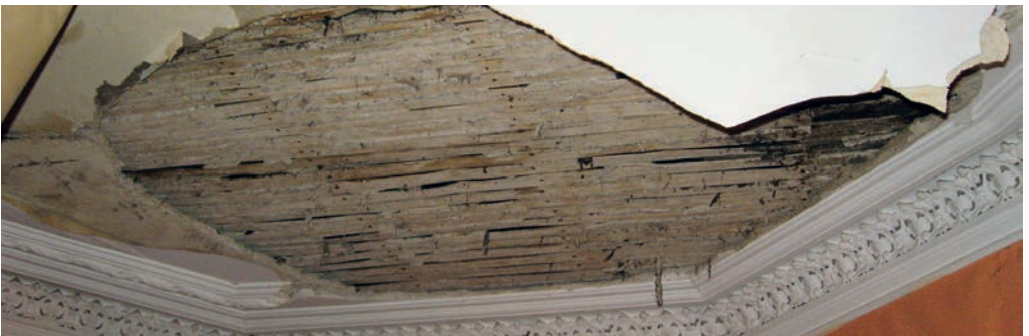
Fig. 3 Water ingress and excess moisture is the most common cause of damage and decay to plasterwork.
