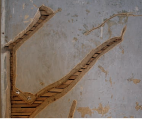
Fig. 7 Loose plaster removed from cracked section of plasterwork - note no requirement to strip out the entire wall lining, patch repair is both achievable and economic.
