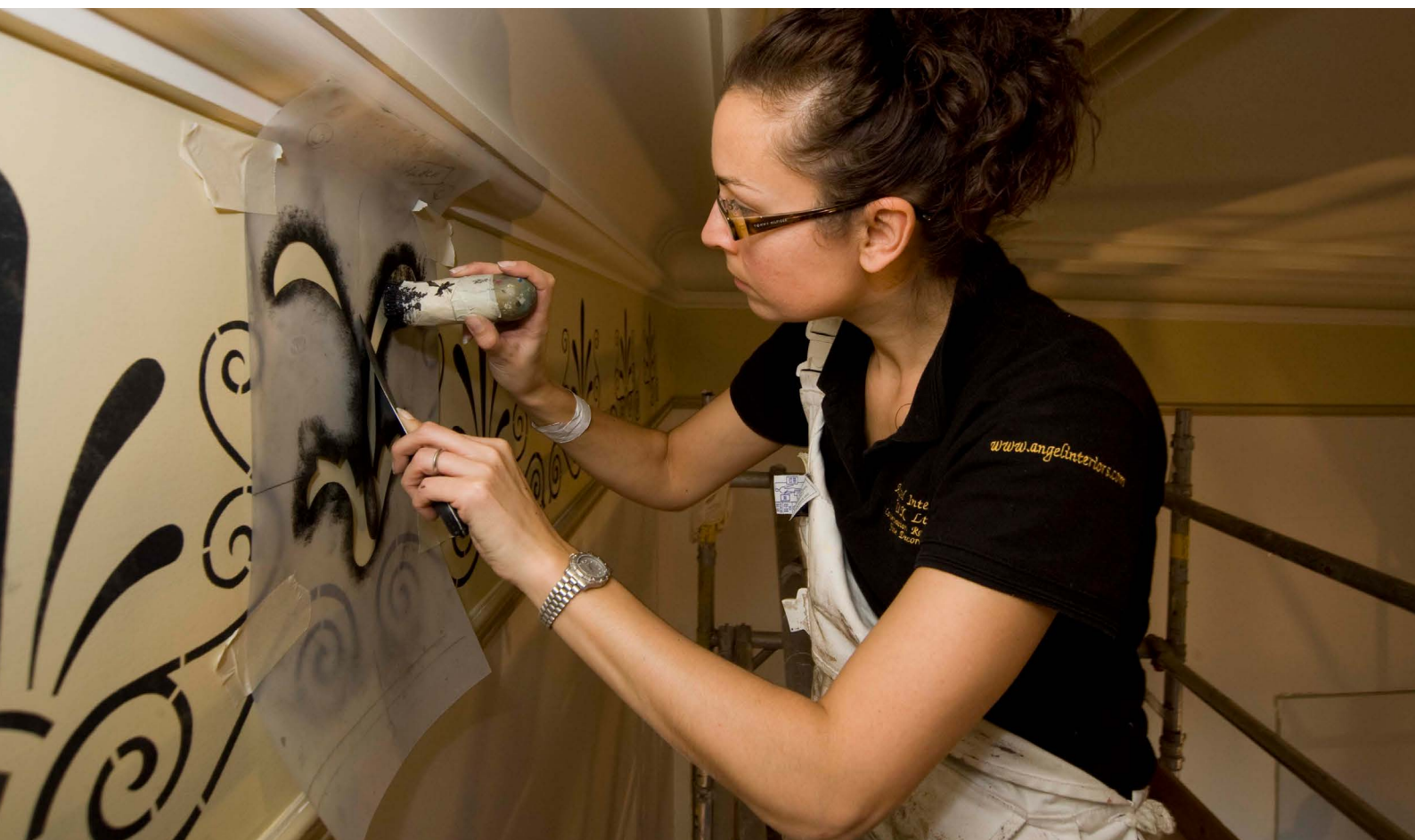
Heritage Bursary Trainee Painter Decorator Lisa Ferguson applying decorative stenciling within a listed building. The placement involved working on a range of historic and traditional buildings and towards a Heritage NVQ Diploma Level 3.
