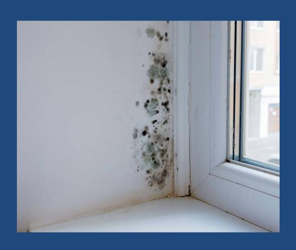
Condensation caused by warm moist air meets a cold surface
