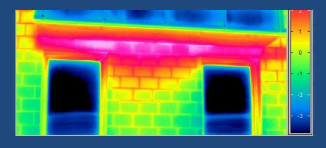
A solid concrete lintel nonrepeating thermal bridge
